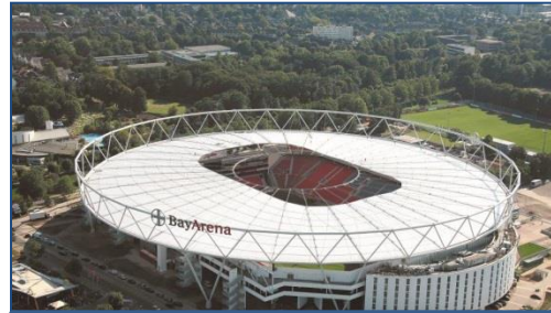
Bay Arena - Germany
