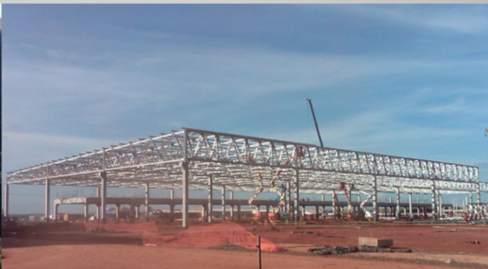
Hyundai Motors - Assembly Shop - 2000 toneladas
