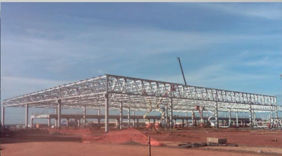
Hyundai Motors - Assembly Shop - 2000 toneladas
