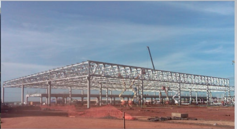
Hyundai Motors - Assembly Shop - 2000 toneladas
