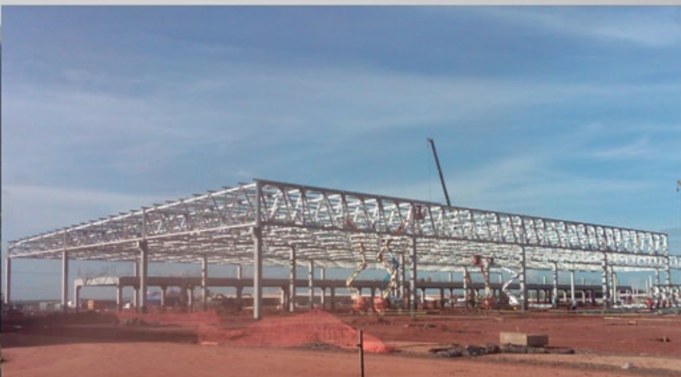
Hyundai Motors - Assembly Shop - 2000 toneladas
